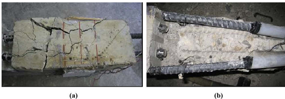
Fig. 10. (a) The cracks after failure in the bonded region of beam F80-U-n1 turned upside down. (b) Intact concrete in the top bar of the beam in beam F80-U-n2.
